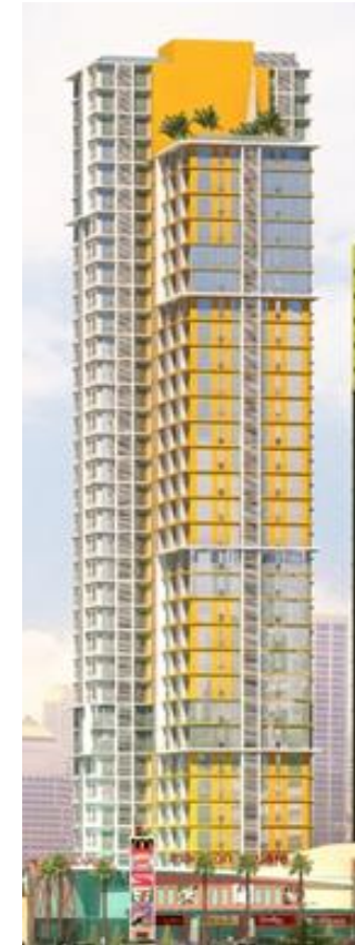
Tower 3: 36-storey TBA
